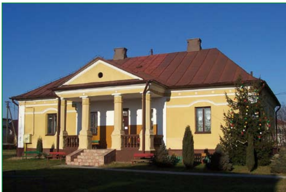
Raniżów – dom pastora (obecnie przedszkole) / former pastor's house (today a nursery school)
